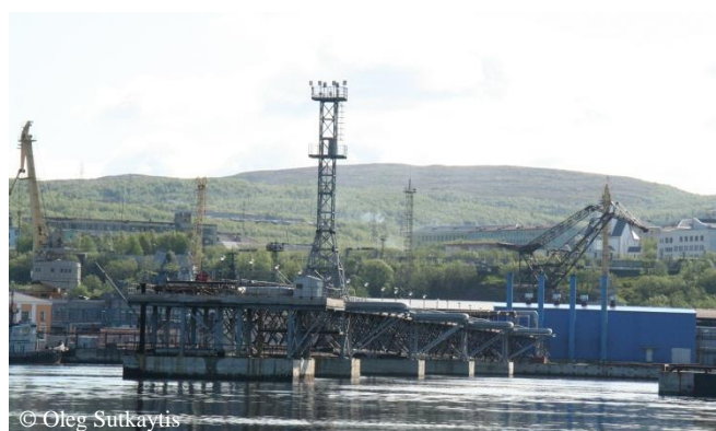
Figure 4.84 The last cargo of export fuel oil was shipped at Polar Terminal in February 2008, after that Trader left the Kola Bay and was decommissioned.
