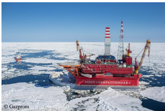
Figure 3.13 The Prirazlomnaya platform was installed in the Pechora Sea in August 2011 and started commercial oil production in December 2013. The first shipment of the Arctic crude oil was done in April 2014. Prirazlomnoye oil field will be in production for 25 years.
