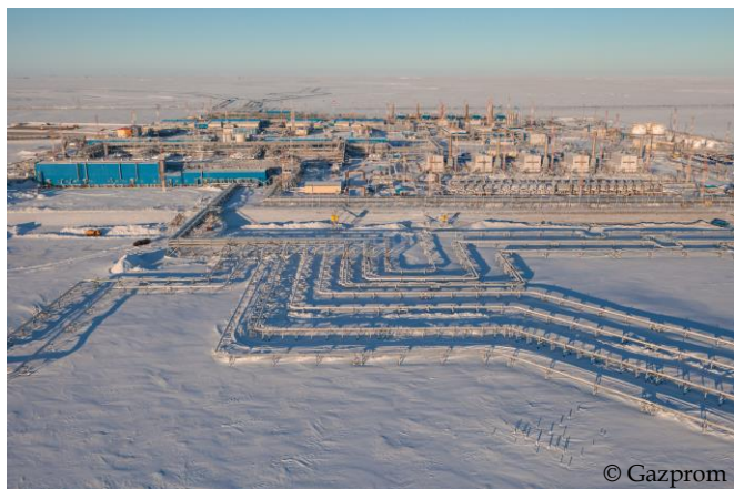
Figure 3.20 Bovanenkovskoye gas and condensate field was put in commercial production in October 2012. More than 38 billion cubic metres of gas was produced at the field in 2014. The maximum gas production level of 115 billion cubic metres per year can be reached in 2017.
