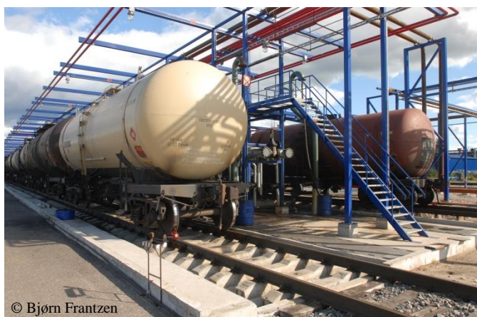
Figure 4.76 Four rail trestles in Vitino port can offload 168 tank-cars with crude and petroleum products simultaneously. The railroad side tracks could receive up to 7 trains.
