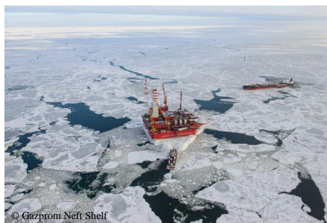
© Gazprom Neft Shelf Figure 4.59 Prirazlomnaya offshore ice-resistant oil-producing platform was delivered to its location in the Pechora Sea in August 2011, and started commercial oil production in December 2013.
