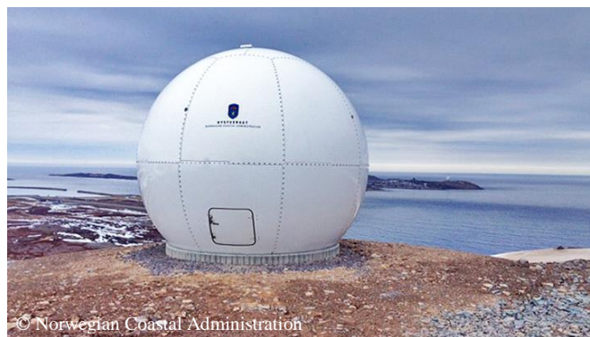
Figure 6.2 Automatic Identification System (AIS) satellite receiving station in Vardø (photo) is a part of the vessel traffic control and monitoring system in Norway.
