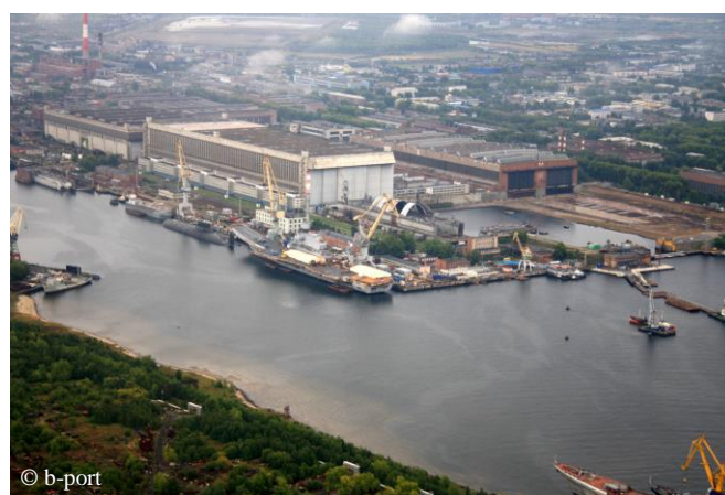
Figure 4.72 The town of Severodvinsk on the White Sea coast with Sevmarsh and Zvyozdochka factories is an important industrial base for the Russian Arctic continental shelf resources development. It was also discussed as possible location for construction of an oil terminal.
