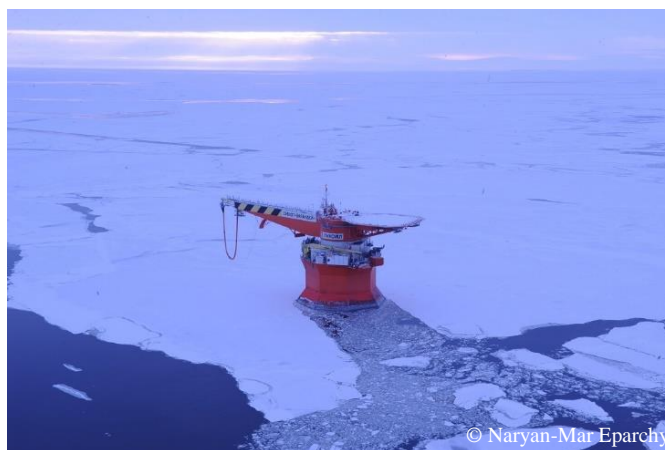
Figure 4.53 Varandey offshore terminal (photo) with the annual capacity of 12 million tonnes is the main oil offloading facility in the Pechora Sea.
