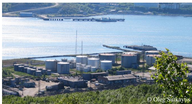
Figure 4.81 The First Murmansk Terminal has been operating the tank-farm of the Murmansk Fishing Sea Port in the Kola Bay since 2005.
