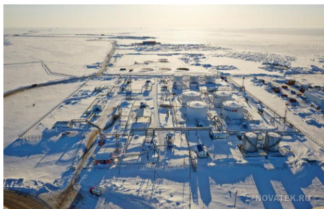
Figure 4.51 Yamal LNG is designed in three phases – three trains to be built. When completed, the plant will produce 16.5 million tonnes of LNG per year.
