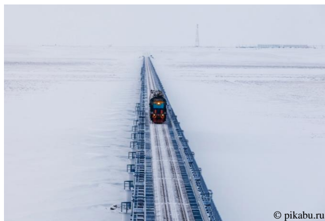
Figure 4.15 A 525-kilometres rail line between Obskaya and Bovanenkovo stations was put on stream in 2010. Photo: 4-kilometres long railway bridge via Yuribey River in Yamal Peninsula.
